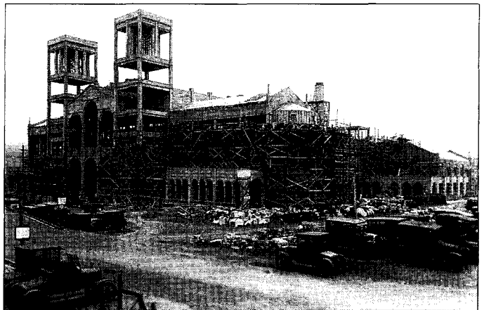
Not the sound of symphony, but of chisel and saw: Royce Hall under construction, 1928.
