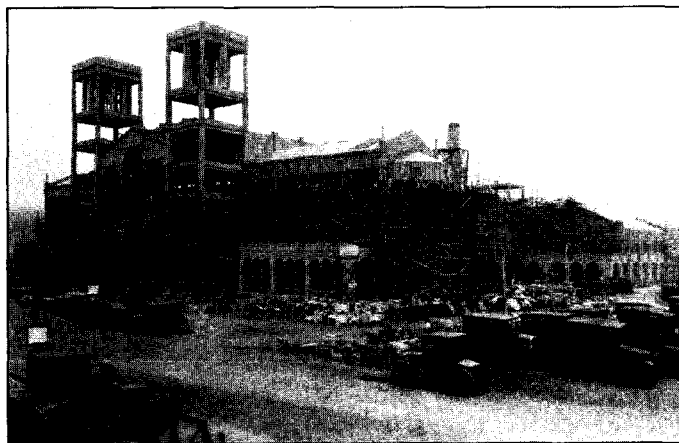
Not the sound of symphony, but of chisel and saw: Royce Hall under construction, 1928.
